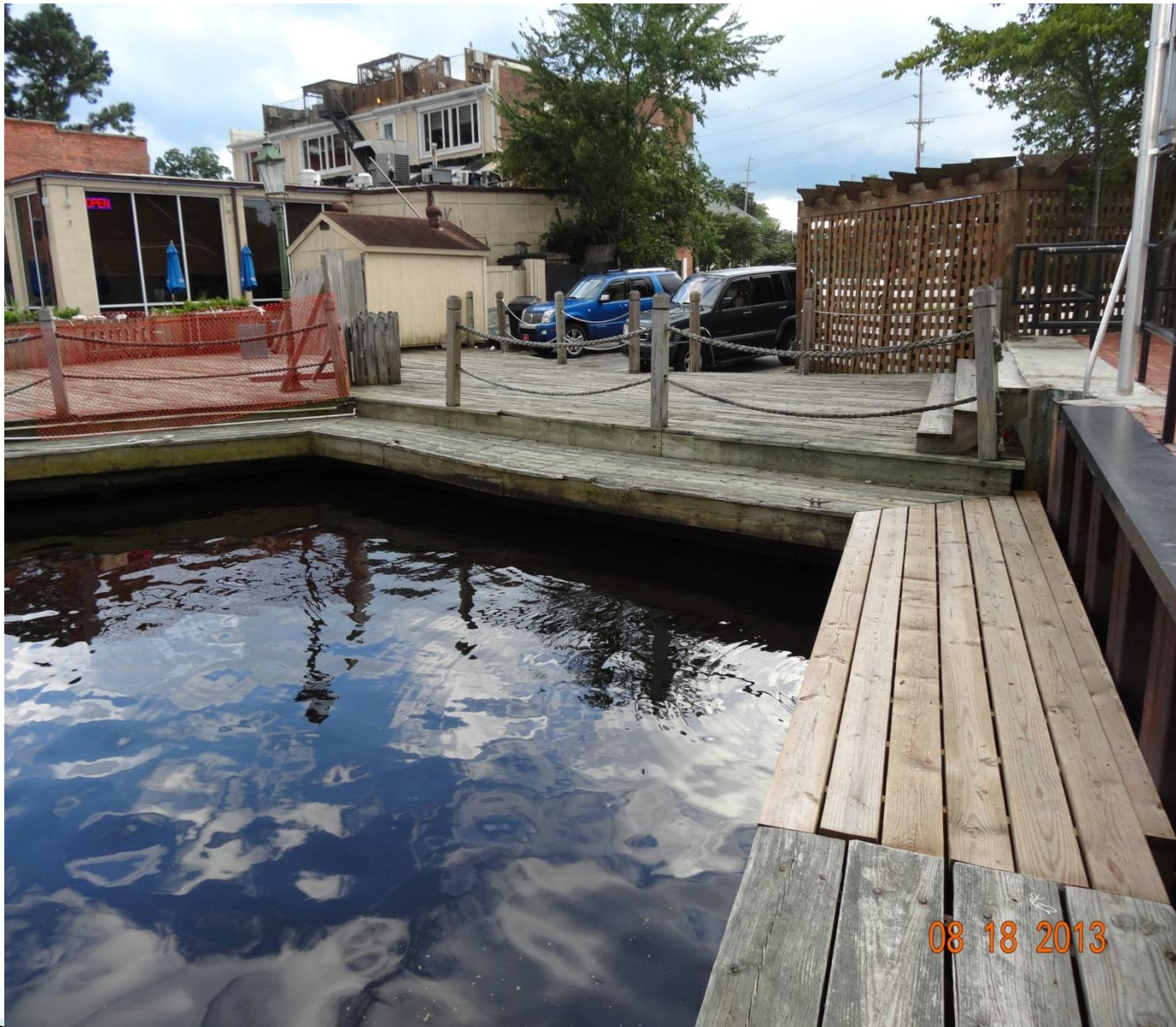
TIBER CREEK STORMWATER MANAGEMENT IMPROVEMENTS 9/23/13
