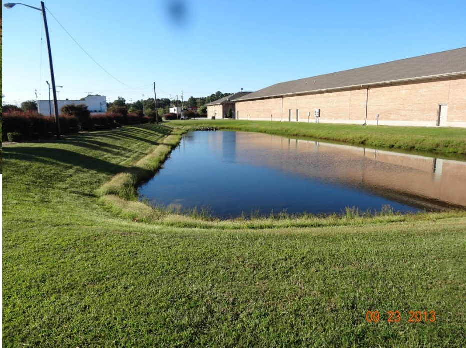
TIBER CREEK STORMWATER MANAGEMENT IMPROVEMENTS 9/23/13
