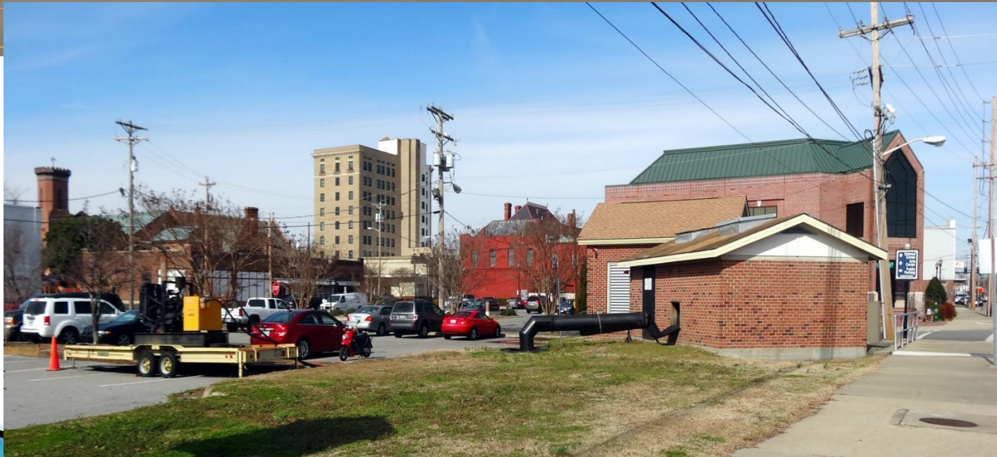
TIBER CREEK STORMWATER MANAGEMENT IMPROVEMENTS 9/23/13
