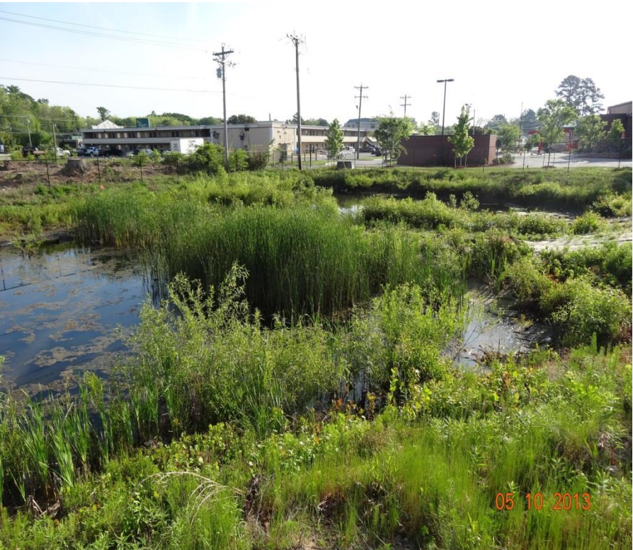
TIBER CREEK STORMWATER MANAGEMENT IMPROVEMENTS 9/23/13
